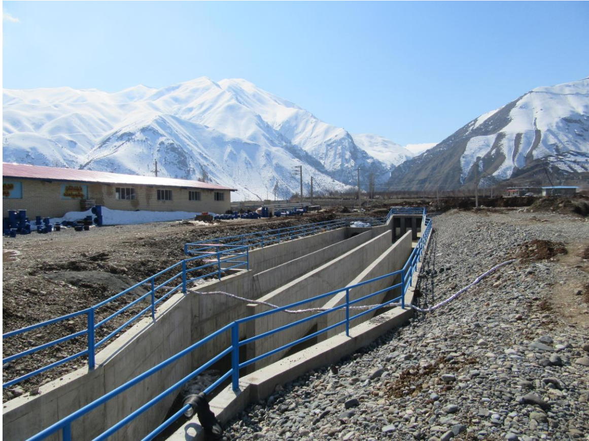
Hydro mechanical Structures Execution of Grade 1 Water Supply Pipes of Badin2 Plain
