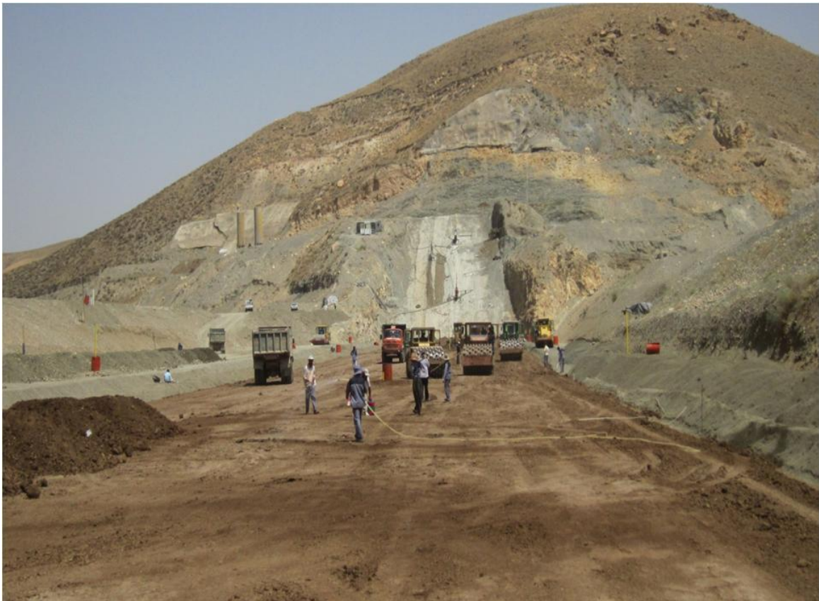
Filling Operation Oshnavieh Earth Fill Dam Construction
