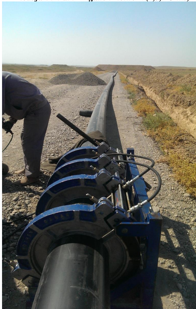
PE Pipe layering Khodafarin Main Irrigation Network (2,3,4 Units)
