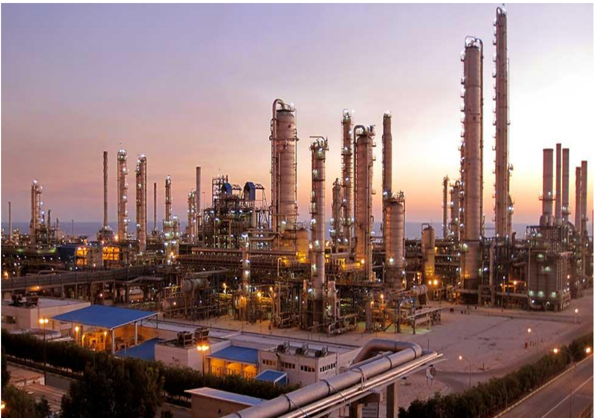
Civil Works of Caspian Sea Republics Oil Swap Project
