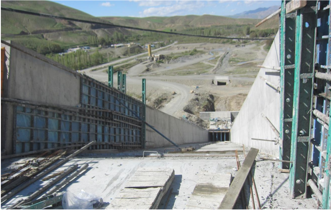
Over Head shoot structure Oshnavieh Earth Fill Dam Construction
