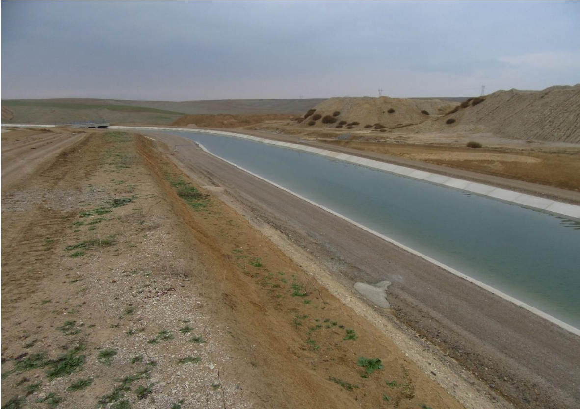
Main channel Khodafarin Irrigation and Drainage Network and Technical Structures 2
