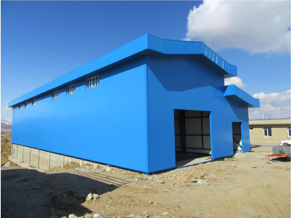
Pomp Station Execution of Grade 1 Water Supply Pipes of Badin1 Plain
