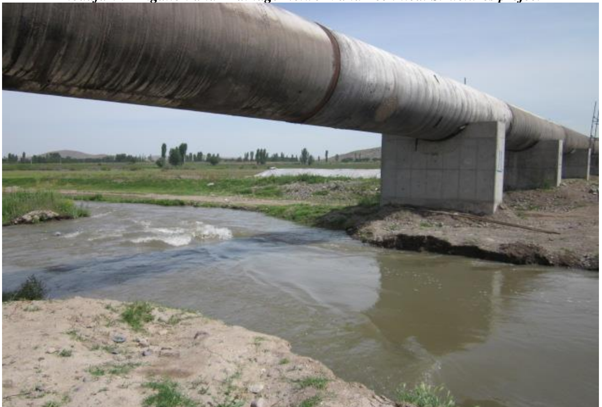
Metal Pipe Syphon Operation Execution of South- North Syphon of Sabalan Dam
