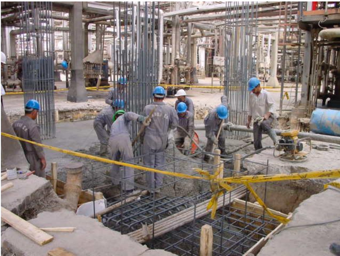
Civil Works of Caspian Sea Republics Oil Swap Project
