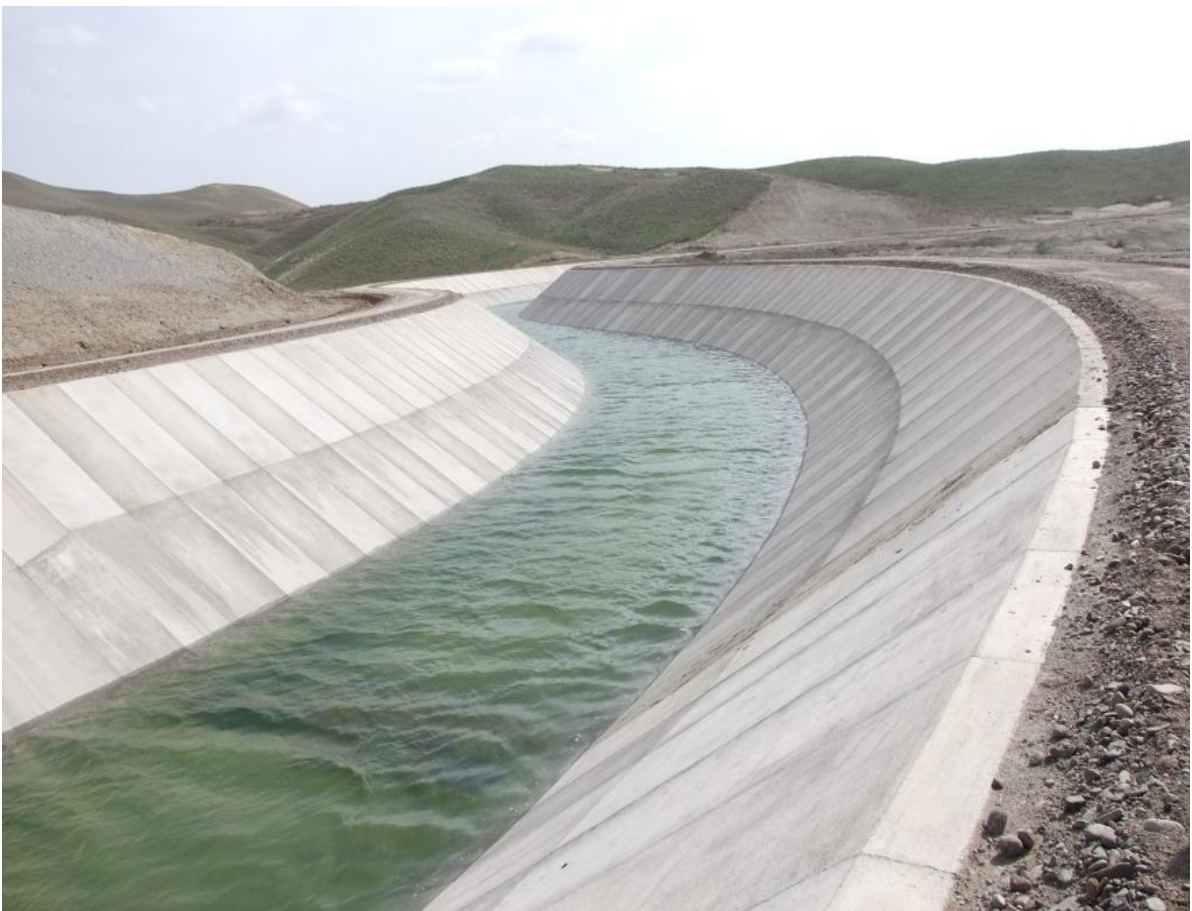
Main channel Khodafarin Irrigation and Drainage Network and Technical Structures project
