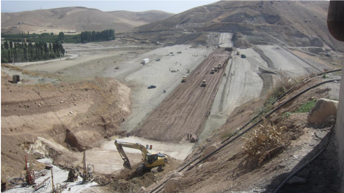
Filling Operation Oshnavieh Earth Fill Dam Construction
