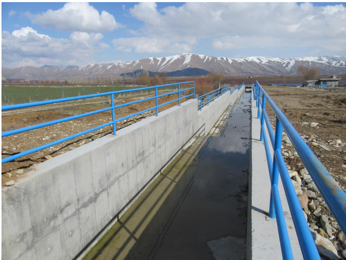
Hydro mechanical Structures Execution of Grade 1 Water Supply Pipes of Badin2 Plain
