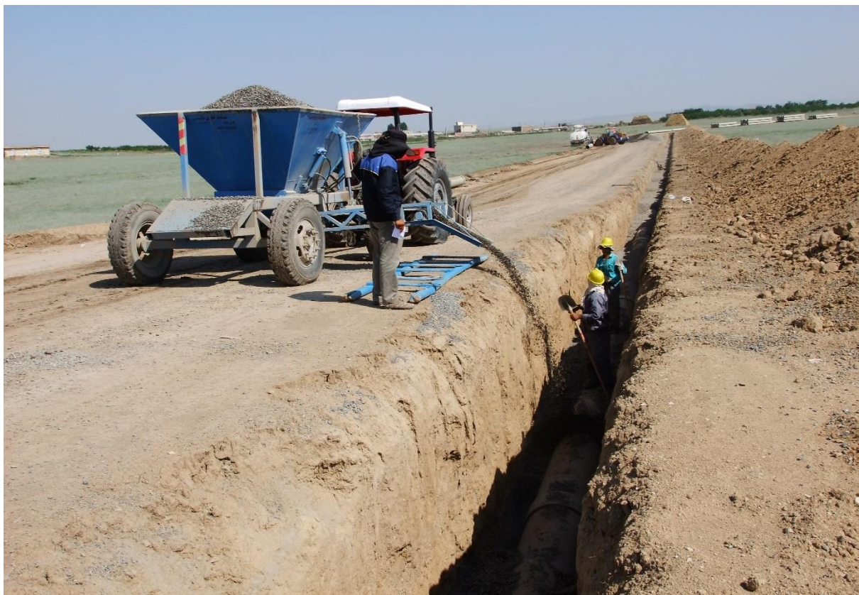
Backfill Operation Khodafarin Main Irrigation Network (2,3,4 Units)
