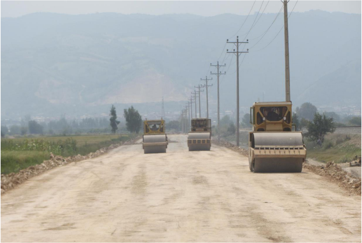
Filling & Compacting Neka Irrigation and Drainage Network project
