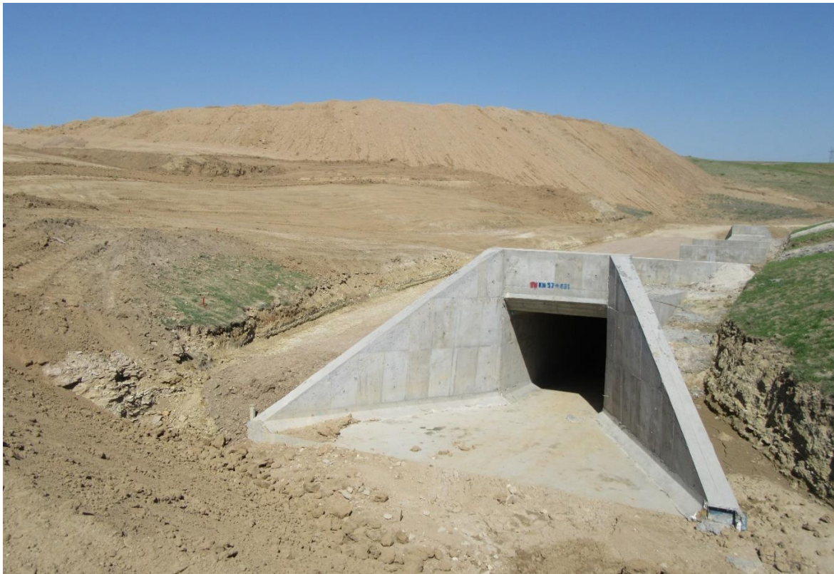
Hydro mechanical Structure Pictures of Neka Irrigation and Drainage Network project
