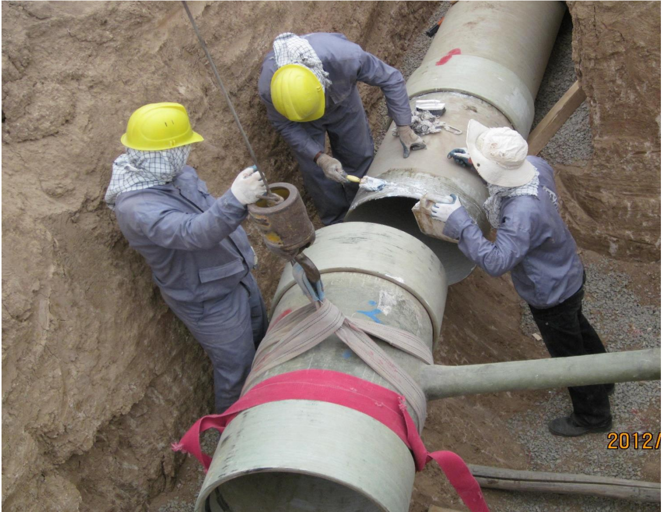
GRP Pipe Layering Khodafarin Main Irrigation Network (2,3,4 Units)
