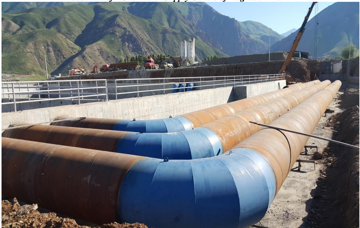
Transition Line Execution of Grade 1 Water Supply Pipes of Badin2 Plain
