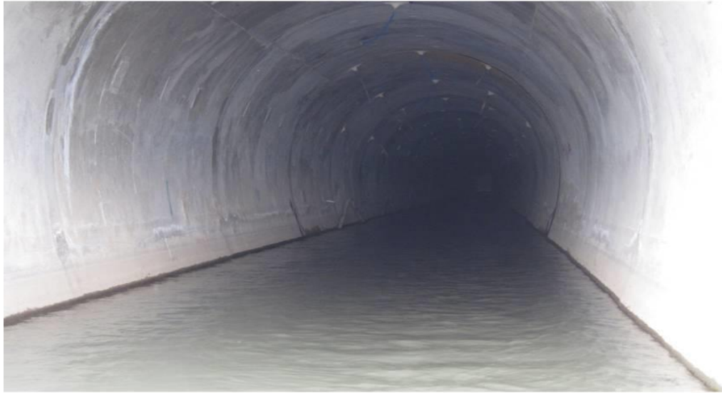
Tunnel Oshnavieh Earth Fill Dam Construction
