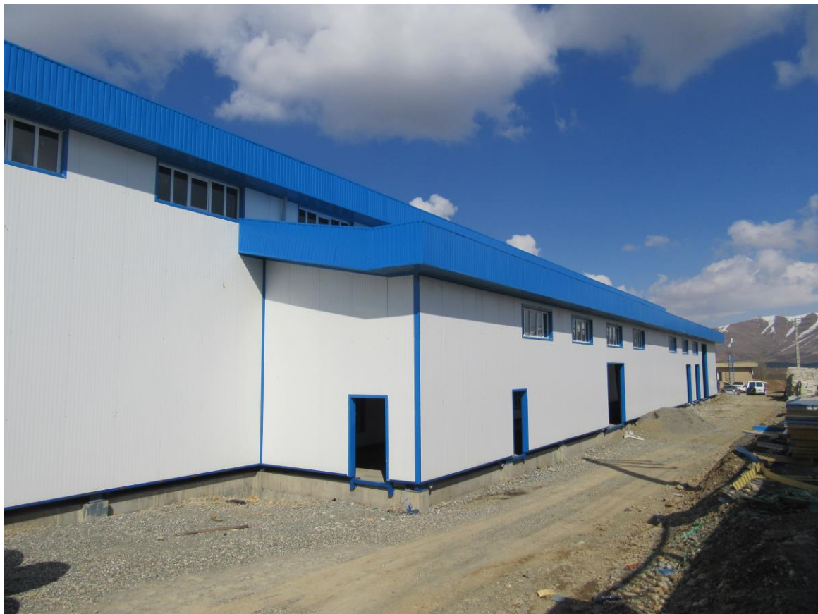
Pomp Station Execution of Grade 1 Water Supply Pipes of Badin2 Plain
