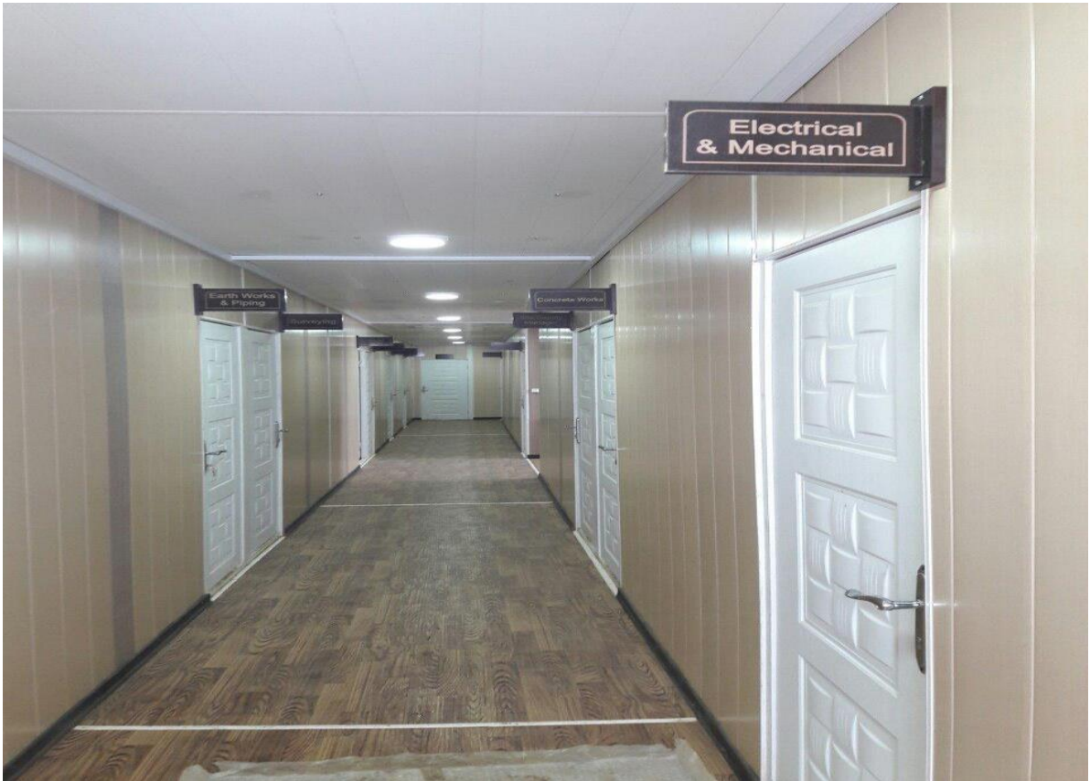
Mobilization & Offices Execution of Grade 1 Water Supply Pipes of Badin 1&2 Plain
