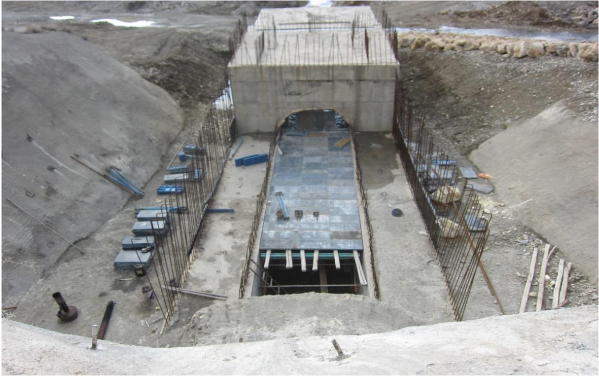
Tunnel Entrance Oshnavieh Earth Fill Dam Construction
