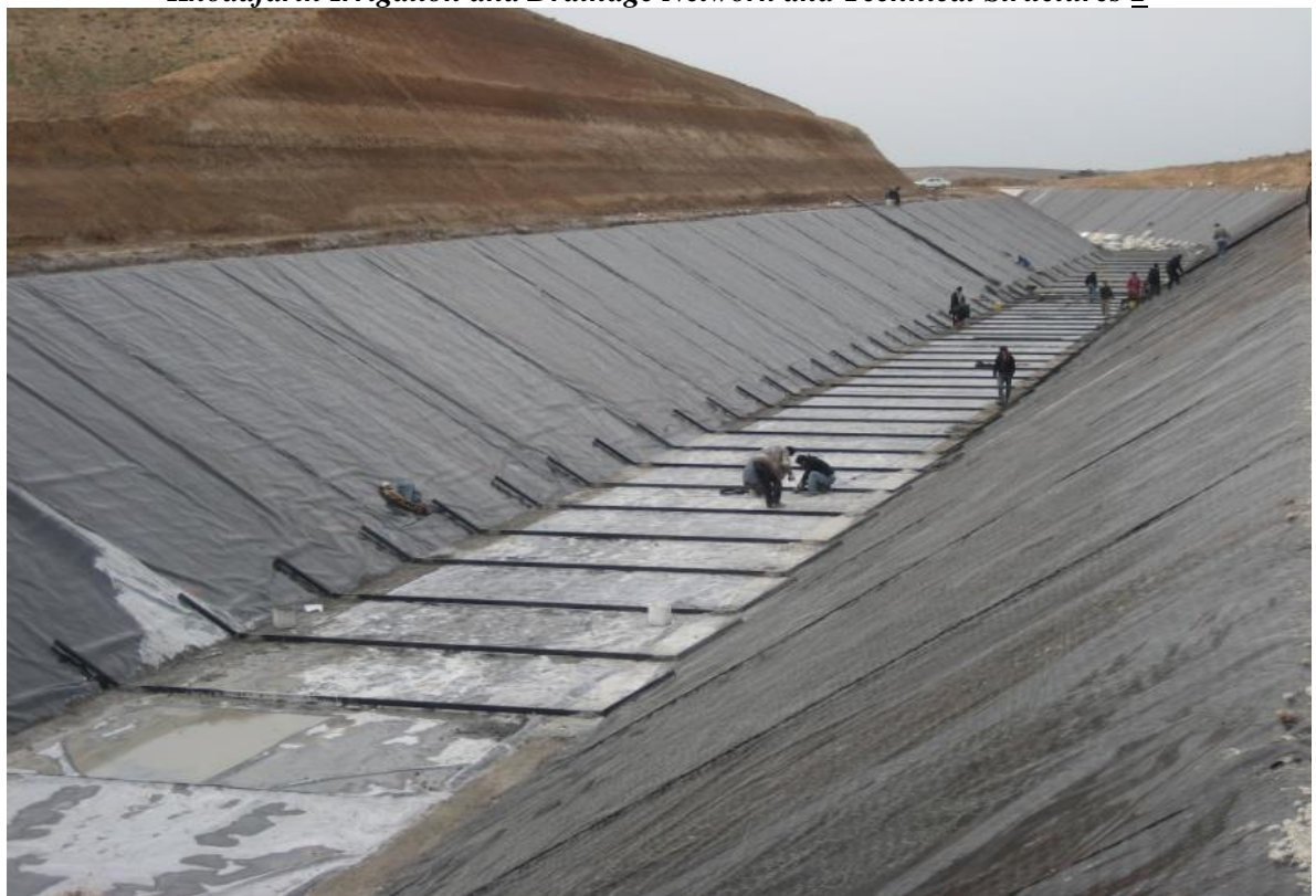
Concrete Lining Khodafarin Irrigation and Drainage Network and Technical Structures 2
