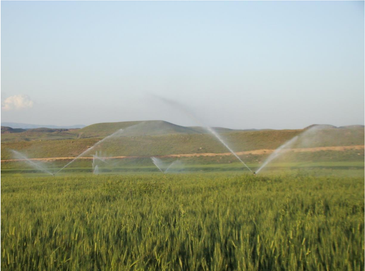
Irrigation Network System Pictures of Downstream Irrigation Network of Sabalan Dam project
