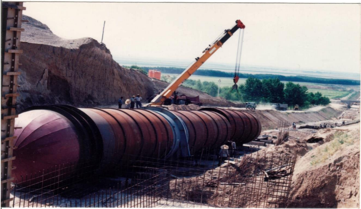
Syphon Structure Khodafarin Power Station
