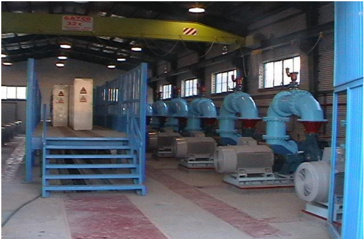
Pump Station Execution of NSP3 Water Supply Canals of Naghadeh Plain
