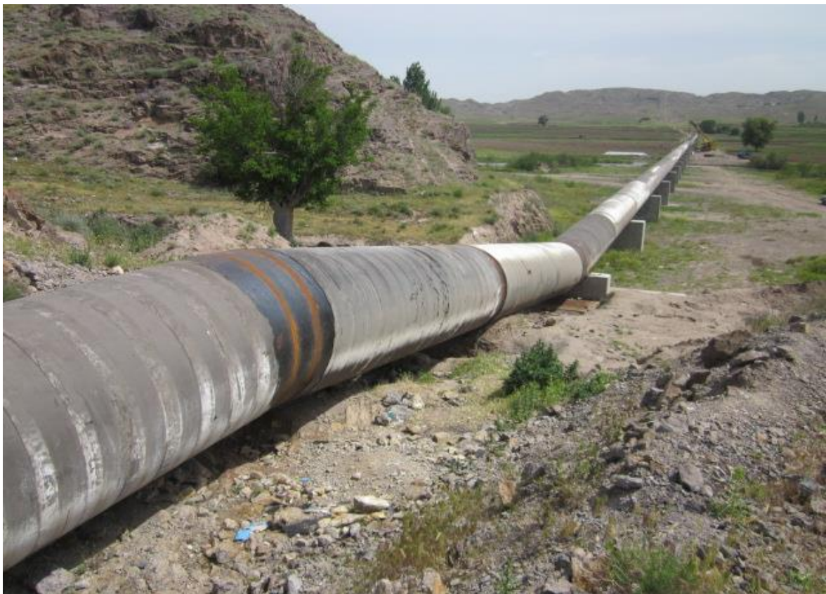
Metal Pipe Syphon Operation Execution of South- North Syphon of Sabalan Dam
