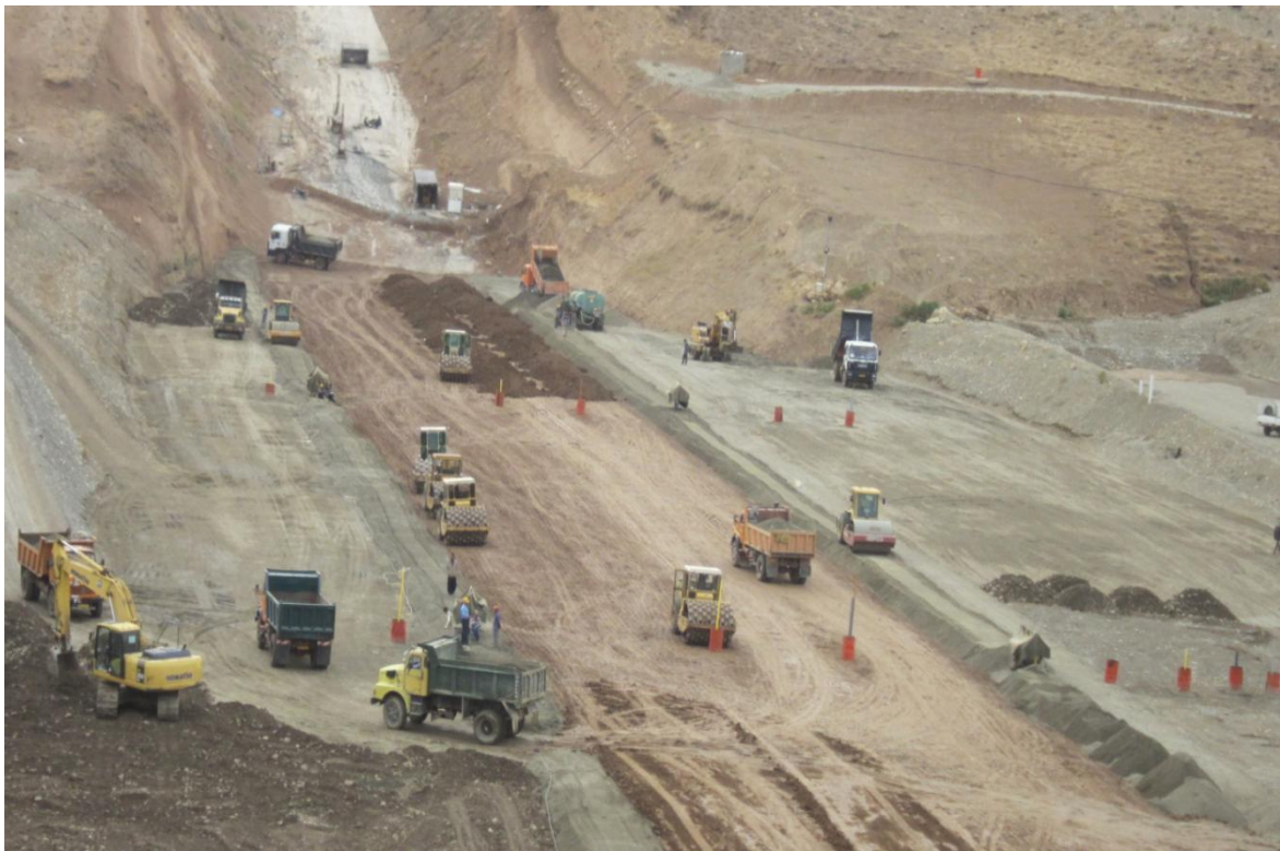
Filling Operation Oshnavieh Earth Fill Dam Construction
