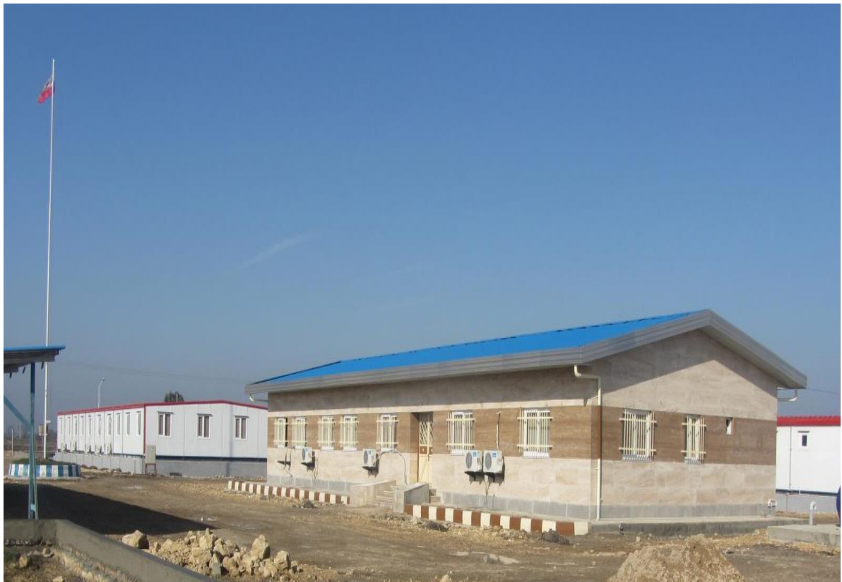
Mobilization & Offices Pictures of Neka Irrigation and Drainage Network project
