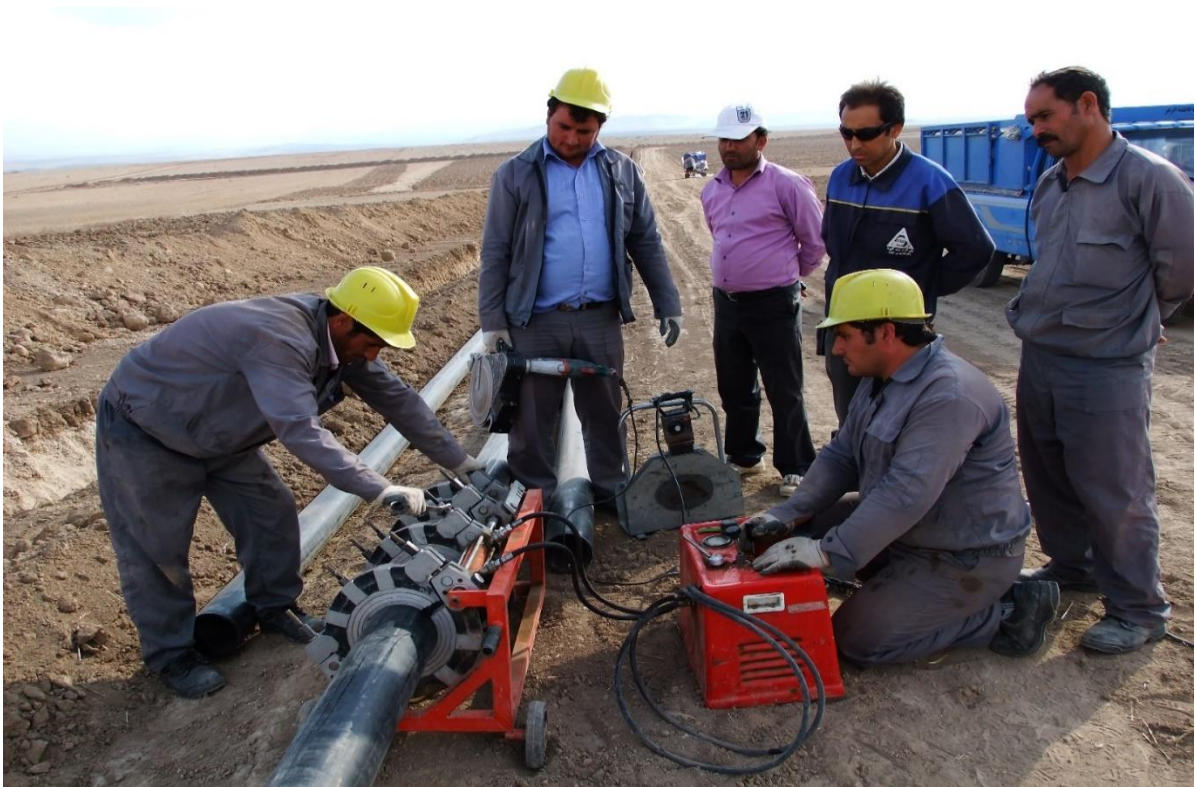
PE Pipe Joining Operation Khodafarin Main Irrigation Network (2,3,4 Units)
