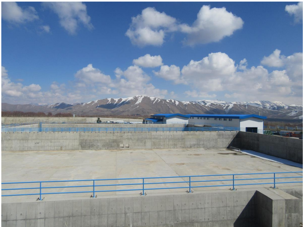
Reservation Structure of Pomp Station Execution of Grade 1 Water Supply Pipes of Badin2 Plain
