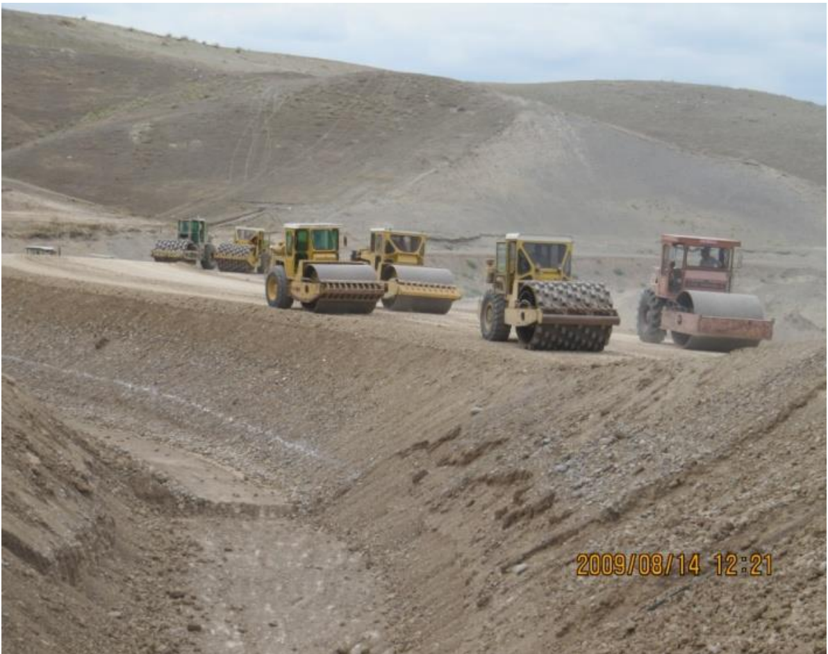
Filling & Compacting Khodafarin Irrigation and Drainage Network and Technical Structures project
