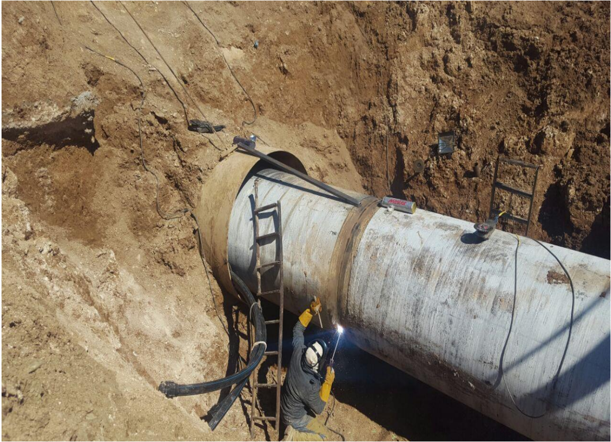
Pipe Jacking Execution of Grade 1 Water Supply Pipes of Badin 2 Plain
