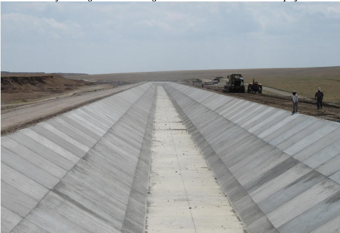
Channel Service Roads Khodafarin Irrigation and Drainage Network and Technical Structures 2
