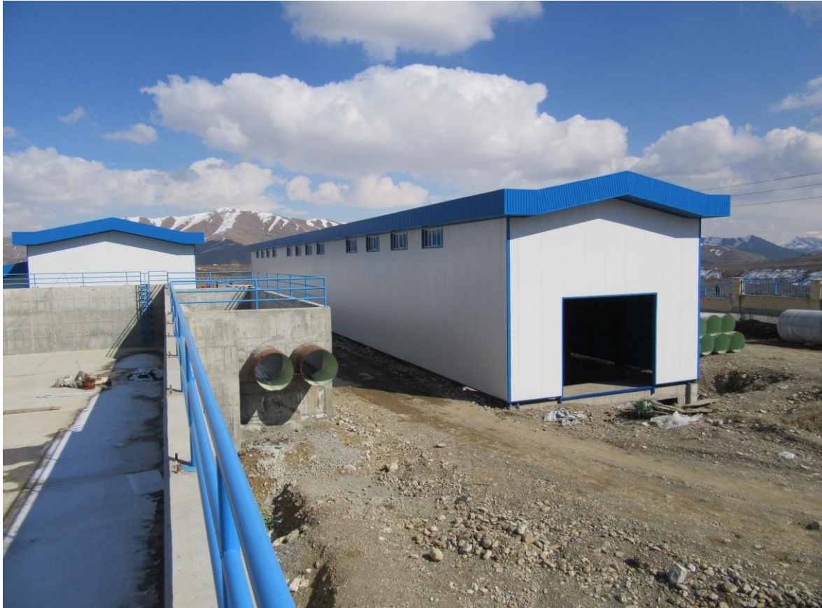
Pump Station Execution of Grade 1 Water Supply Pipes of Badin2 Plain
