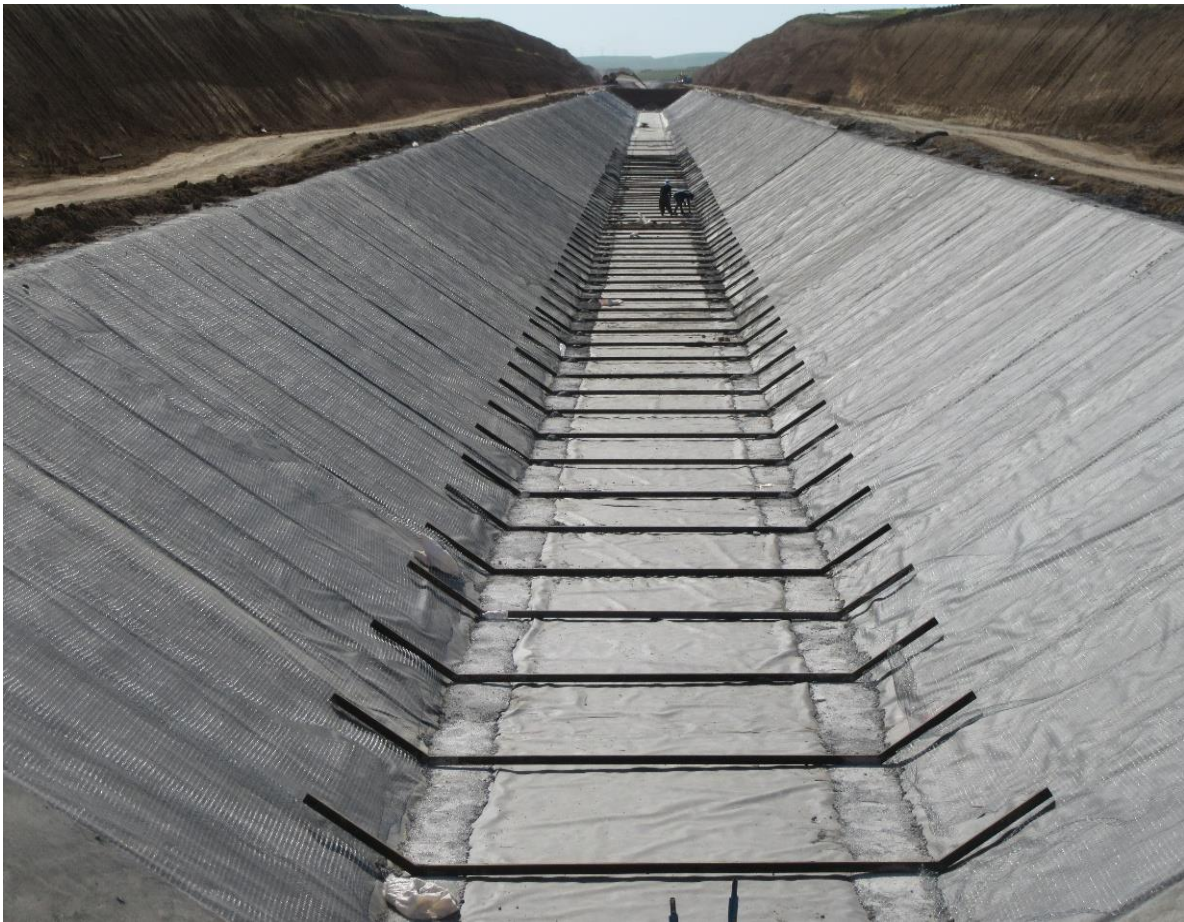
Concrete Lining Khodafarin Irrigation and Drainage Network and Technical Structures project
